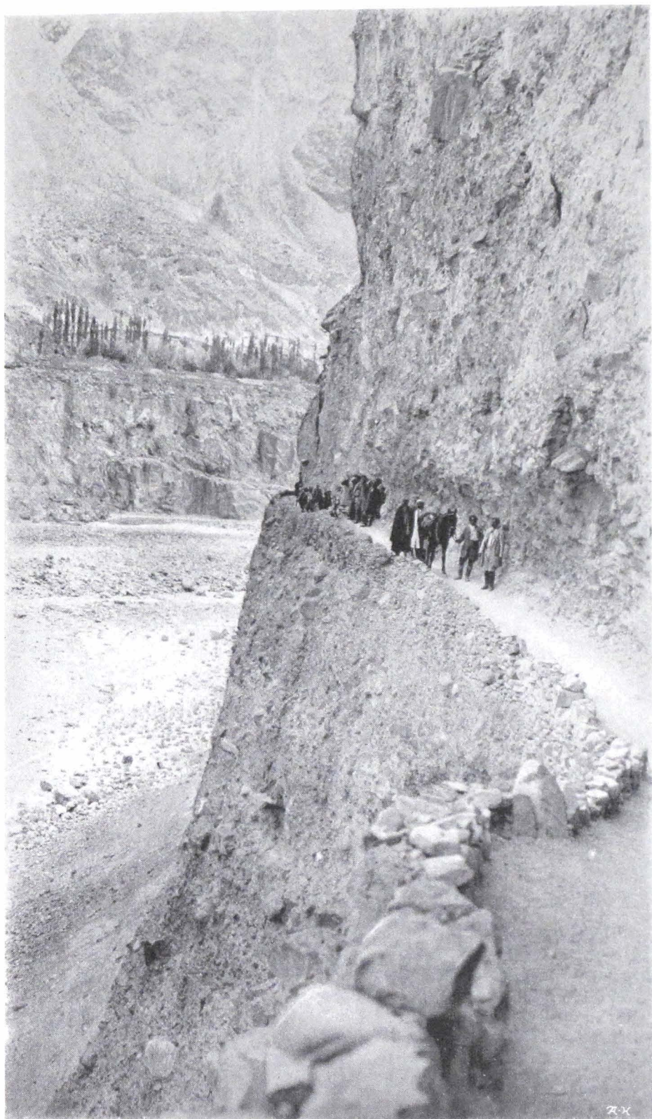
The road between Chalt and Nilt. The Hunza River below. Looking Eastwards.
